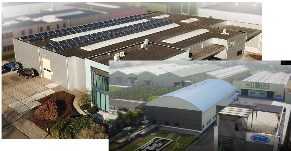
▲ The solar panels installed on the rooftop of our Taiwan and Europe company
